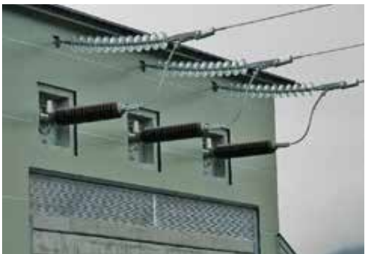
› Indoor/outdoor wall-bushing in a distribution substation.
