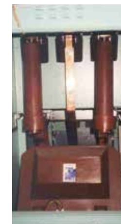
> Support type voltage transformers with fuse VCT type.
